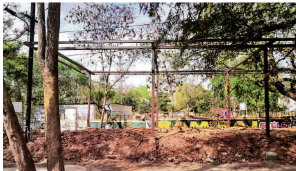
Construction works for the model road project in progress on Race Course Road in the city on Friday.
